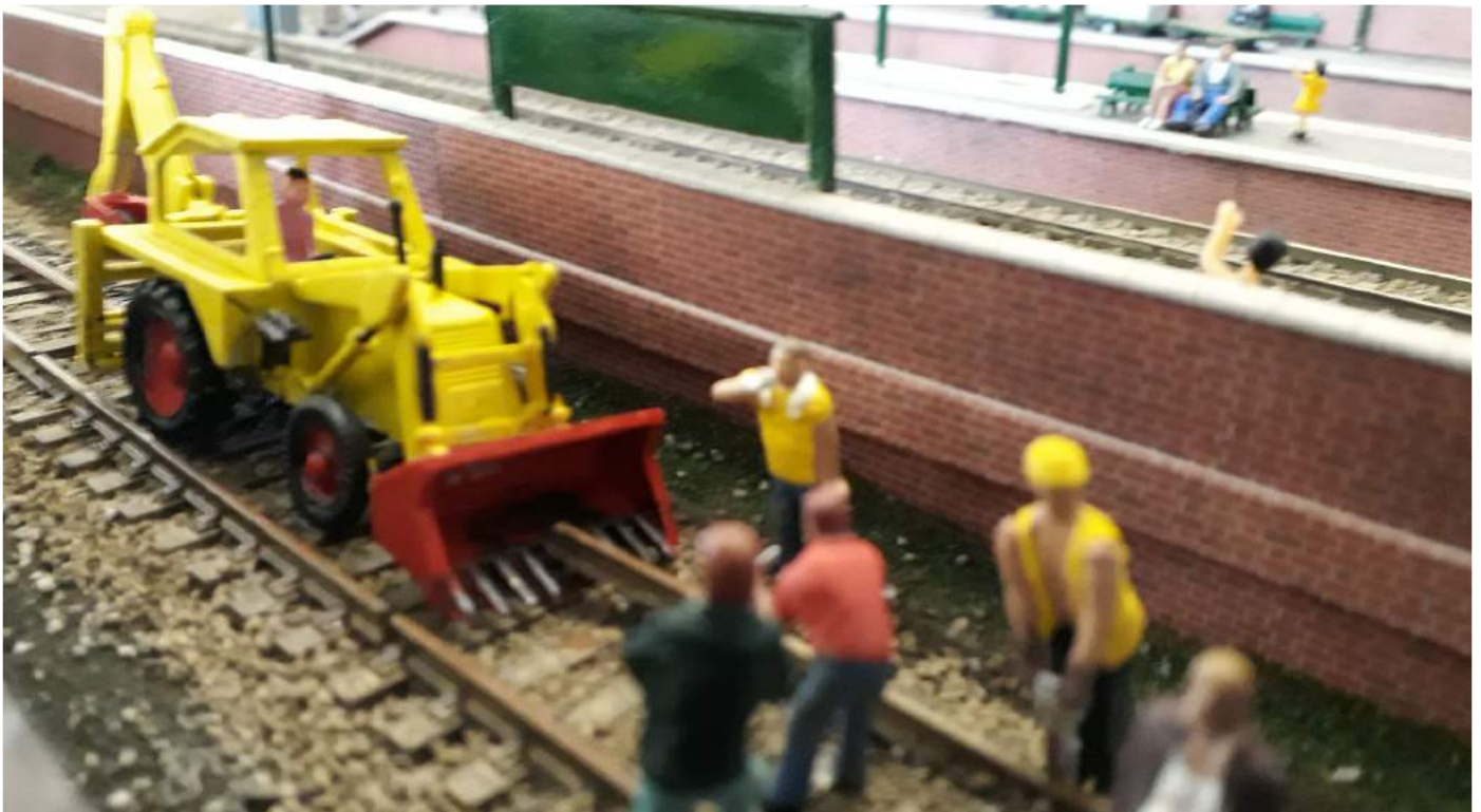
Removing redundant track
