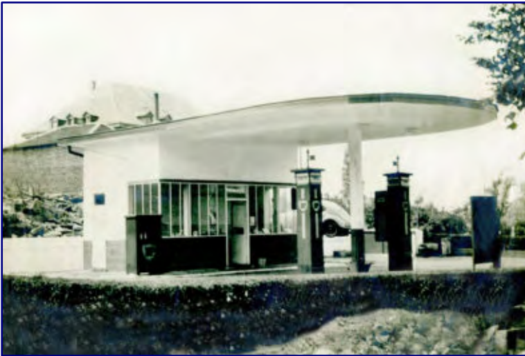
Hand pump columns, here at a BP station, disappeared quite quickly after the Second World War and made way for more modern types of construction. Photo: Sammlung Ulrich Biene
