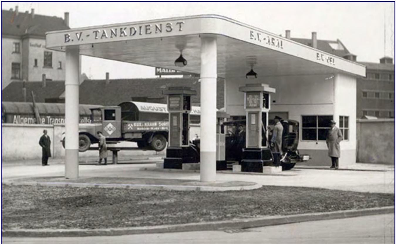
An early representative of the large filling stations is this BV-Aral station in 1939, with its high hand pump columns and the still outdoor lifting platform for work on vehicles. Photo: Historisches Archiv BP/Aral
