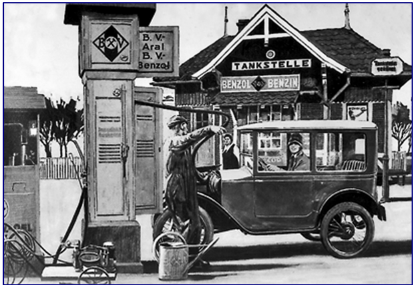
This BV-Aral petrol station from 1924 gives an idea of the first stations that emerged in this decade. Diesel fuel was not available there at that time. Photo: Historisches Archiv BP/Aral
