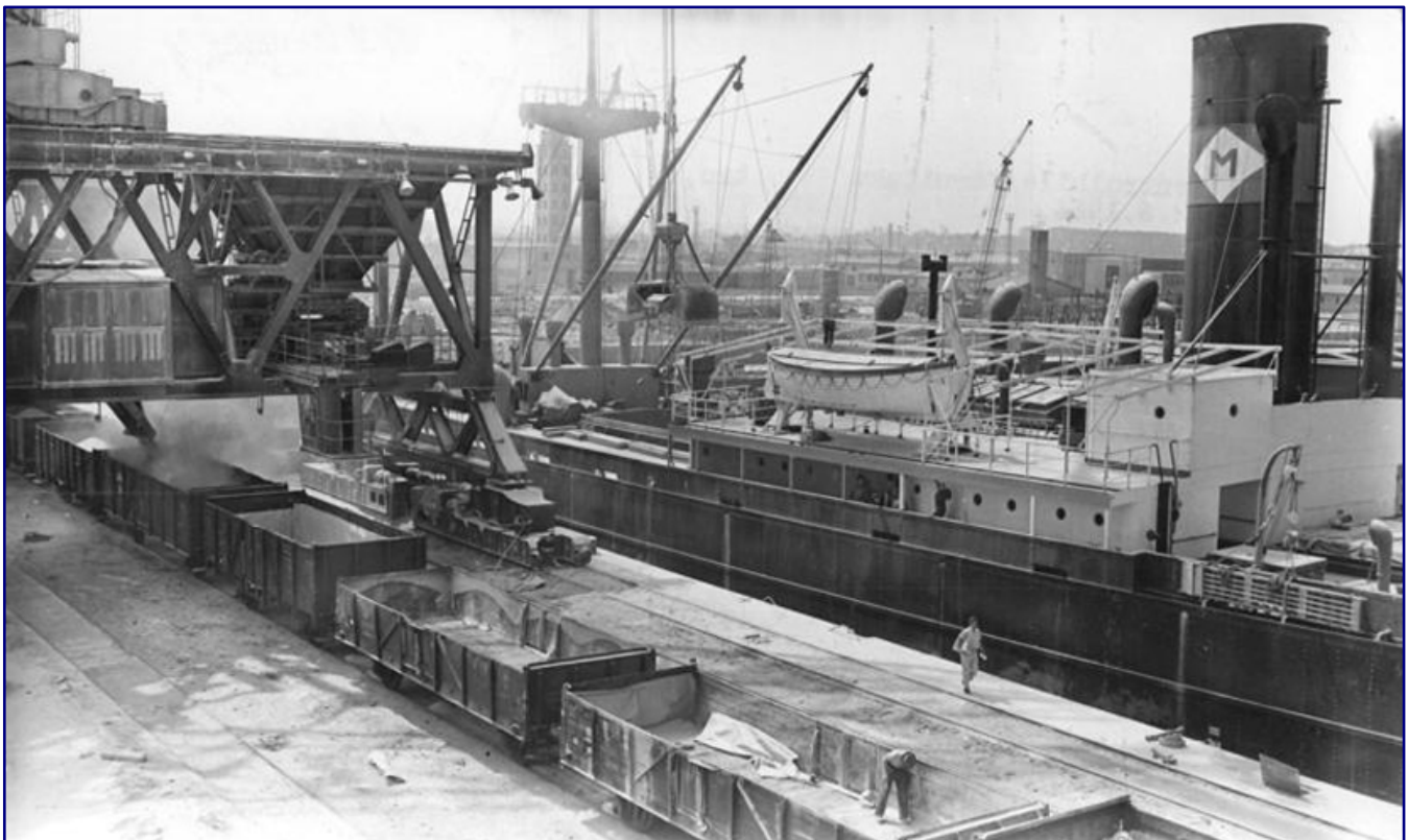
Open freight wagons have always played a large and important role in the railway. Here, in Rostock Überseehafen (Overseas Harbour) on 22 June 1964, you can see, among other things, specimens from the former Lin type. Photo: Bundesarchiv, Bild 183-C0622-0004-003 / CC-BY-SA 3.0
