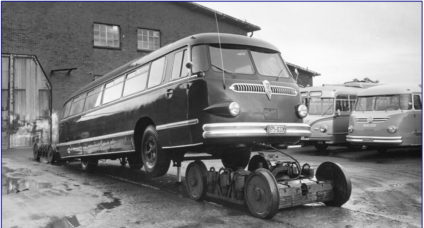
The test vehicle is used to illustrate the operation of the hydraulic lifting system for the works photographer. One after the other, they lift the bus at the front and rear so that the trolley can be pushed underneath. The two prototype rail cars with the different track block brakes are used here again as a demonstration object. Photo: Factory photo NWF, Archive Bernd Coldewey
