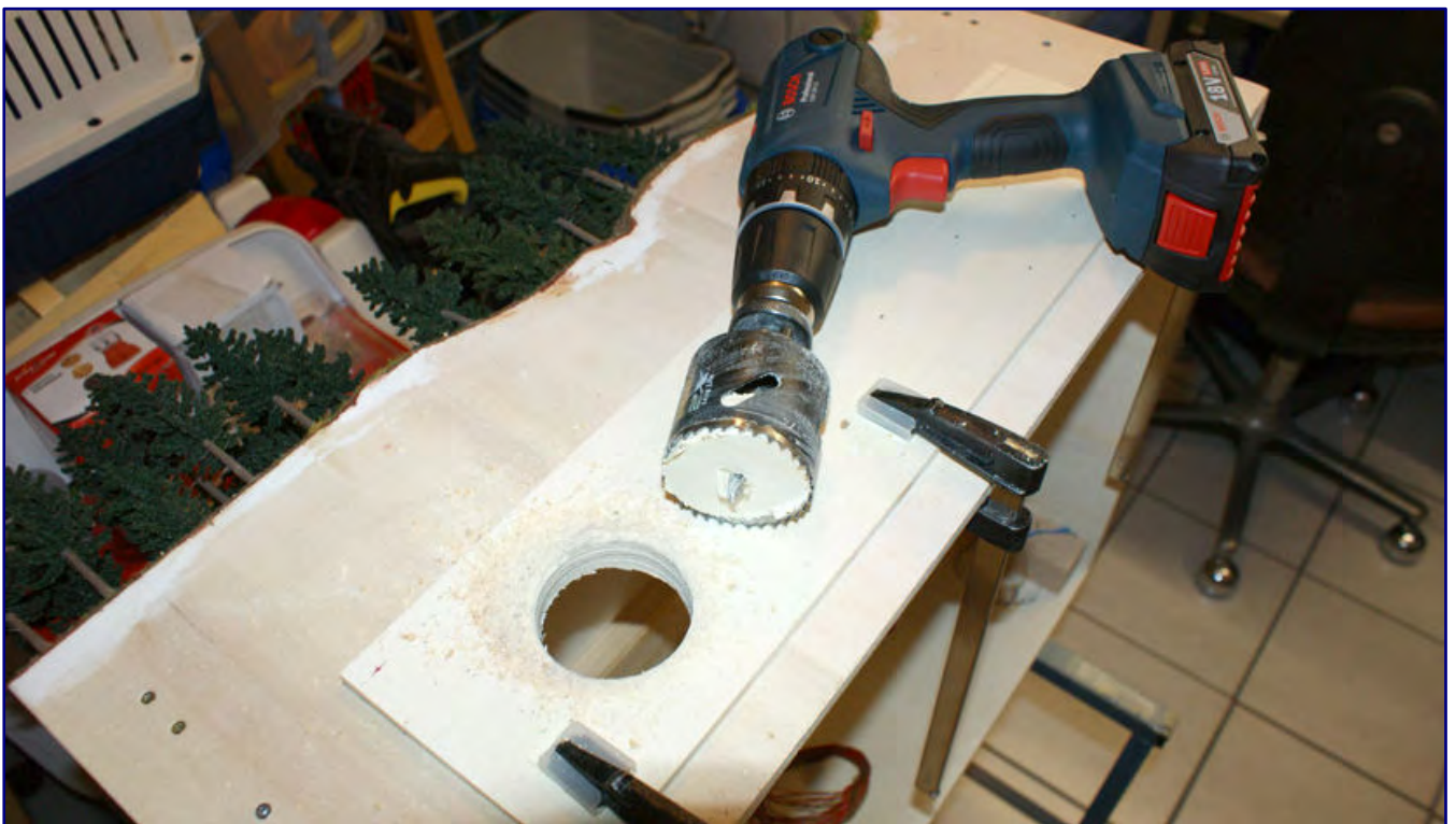
The plywood panel, later to be mounted underneath the backside of the diorama, is first placed on top, aligned and fixed with clamps. The holes are then drilled with a cordless drill, first with a hole saw, and then with Forstner drill bits of two different diameters.
