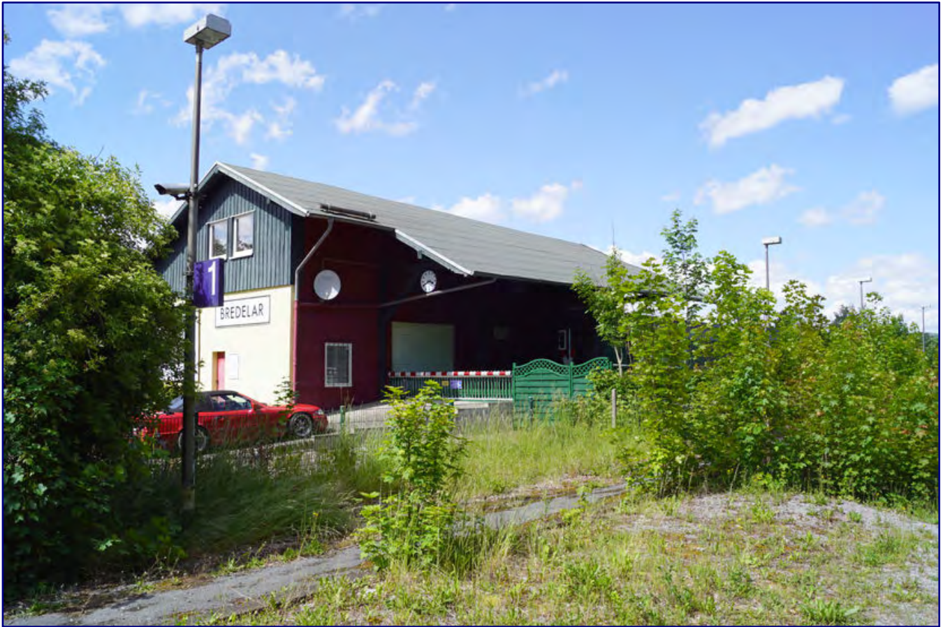
At Bredele station, the single-track dismantling between Brilon and Warburg is particularly easy to follow: Today only one stop with one track, the station building, which has long been privately used, is conspicuously far away from it in June 2020. Photos: Märklin
