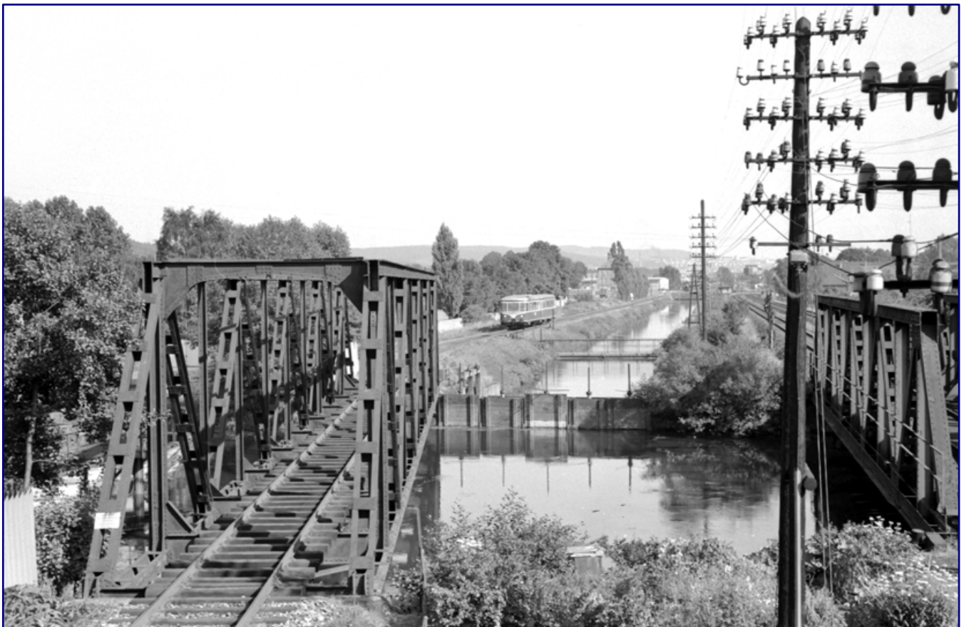
The VT 5 of the Ruhr-Lippe Railway (predecessor company of RLG) was taken up on 1 September 1962 on the Neheim-Hüsten - Arnsberg line at the Röhrbrücke near Arnsberg. There was still road scooter traffic on this line until 1994. On the right of the branch line you can see the double-tracked line of the Oberen Ruhrtalbahn (Upper Ruhr Valley Railway). Photo: Gerd Wolff, Eisenbahnstiftung
