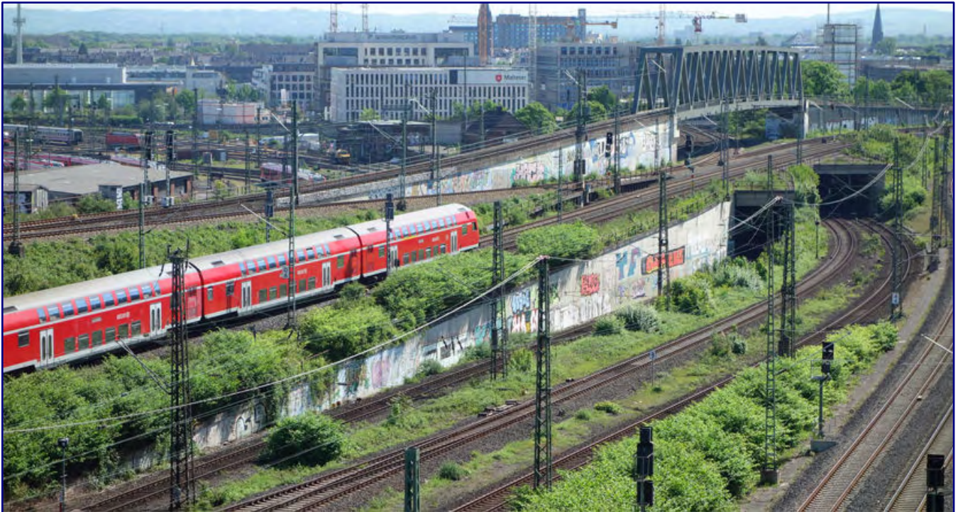
We often find ramps and overpasses in areas close to cities where various railway lines branch off. The example here shows a scene from Köln (Cologne).
