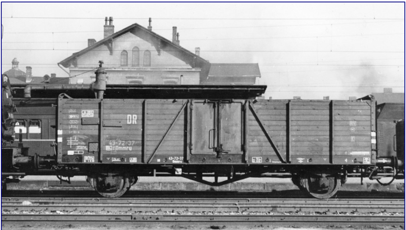
After the Second World War, the wagons were scattered all over Europe and were partially rebuilt. The Ommru coach 43-72-37 remained with the Reichsbahn in the DDR and is shown there in 1959 in its original condition. Photo: Gerhard Illner, Eisenbahnstiftung
