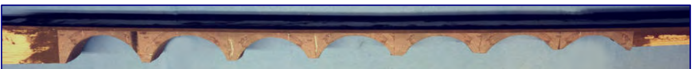
In the centre of the pier, the butt edges are not to be aligned exactly: they will still be covered by a brick masonry support later on.
