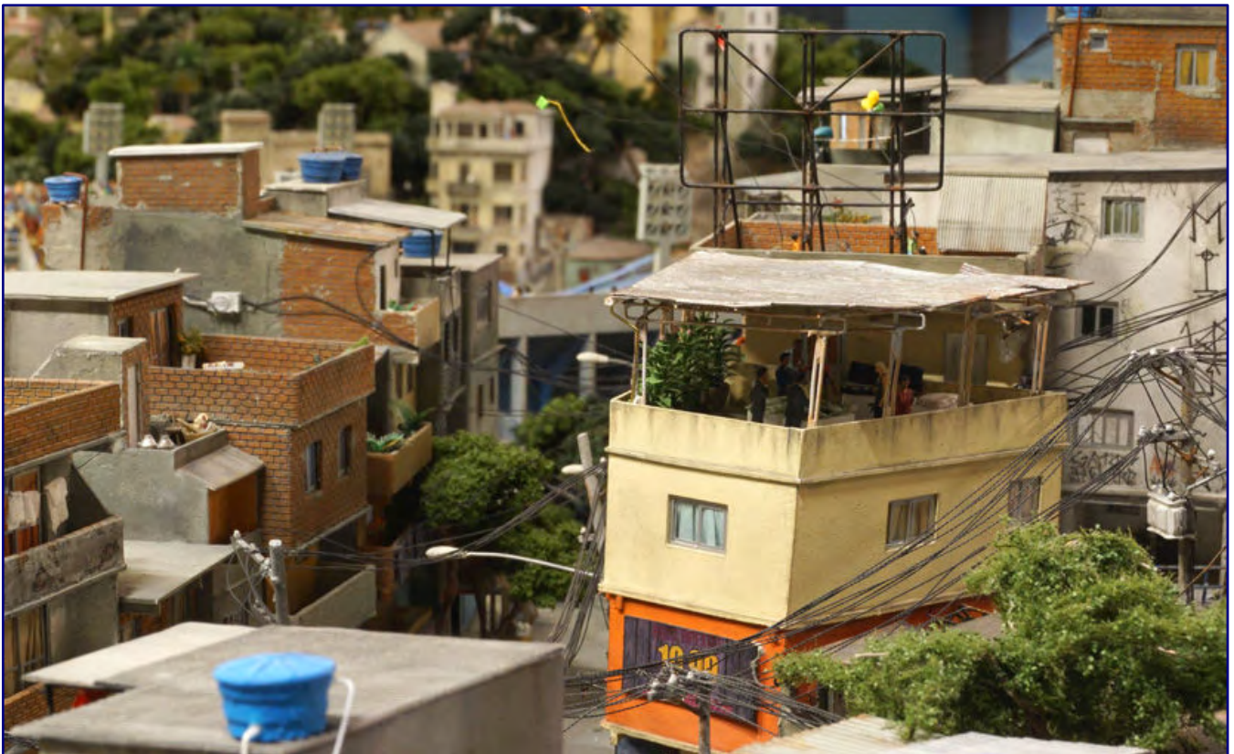
Life in the favelas seems to be characterised by rooftop parties (top photo) and massive drug dealing on the roof terraces (bottom photo). Typical is also the “cable clutter” of the power supply lines, which can also be partly seen on the right of the photo. Brazilian joy of living is represented by the carnival in Rio de Janeiro, characterised by samba rhythms and dazzling costumes (photo on page 40). The opening ceremony in Hamburg was no exception.
