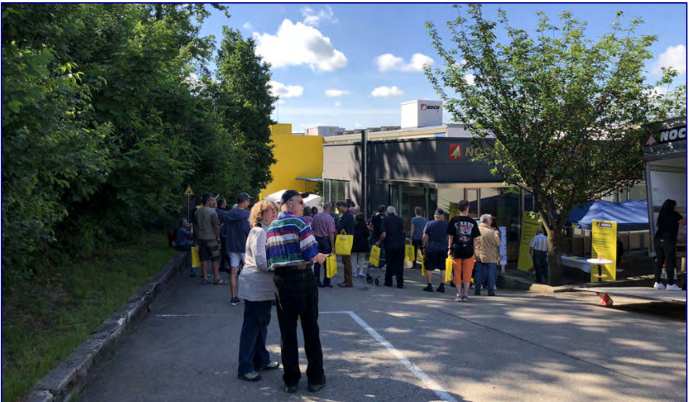
Facing away from the road are the administration and production buildings. The automated small parts warehouse, which can be seen in yellow in the background, is very interesting for visitors. Photo: Noch
