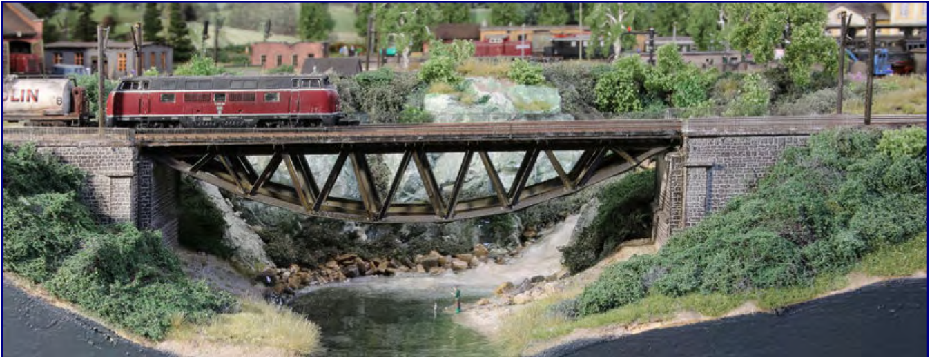
The fish-belly girder bridge by Hack is one of the “highlights” of this Z layout. Although all tracks are at one level, the bridge suggests a mountainous landscape.
