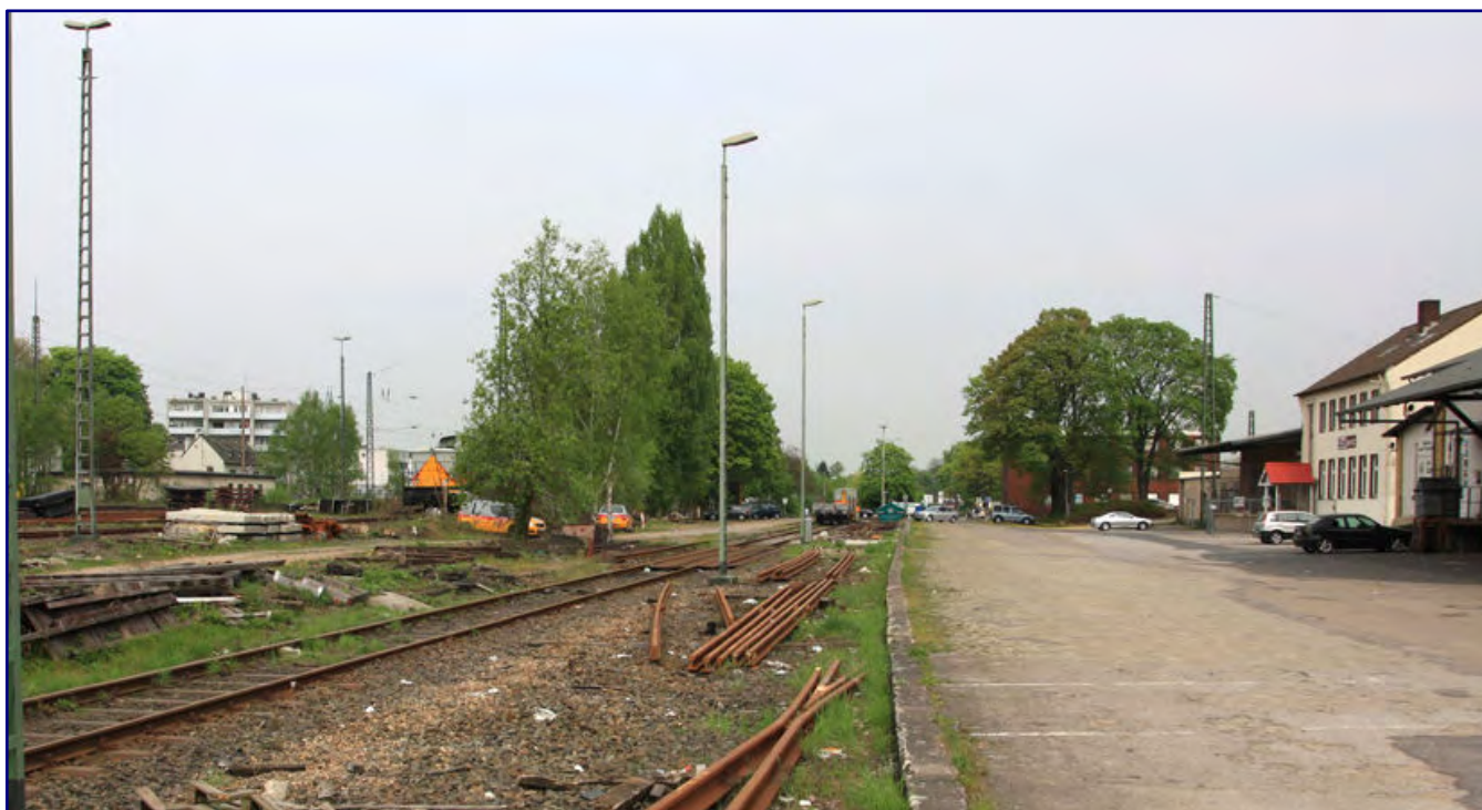
The central signal box had been out of service for several years when this photo was taken in 2013 (top photo). The remains of the open-loading access at Opladen station (bottom photo).
