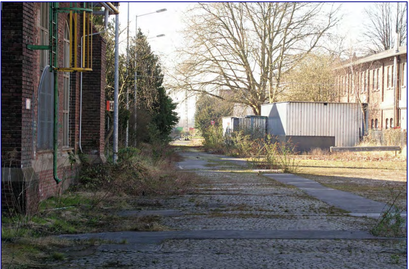
View into the old car shed 1 of the repair shop, even the 24m car transfer table had been dismantled long ago (photo above).
