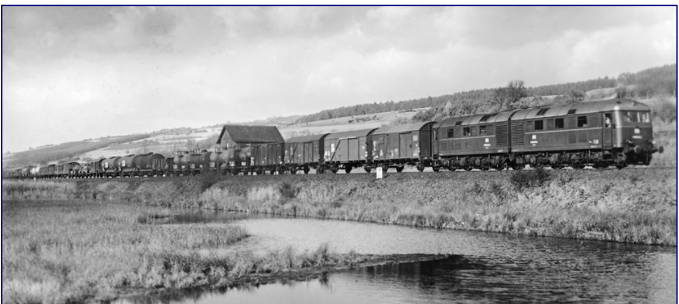
Heavy goods trains were their field of activity: The driver of V 188 001 a/b receives the braking slip before the journey starts (photo above). V 188 002 a/b is on the north-south line between Mottgers and Gemünden near Mittelsinn on 14 September 1959 (photo below). Photos: Peter Pfister (photo above) / Carl Bellingrodt, Eisenbahnstiftung (photo below).
