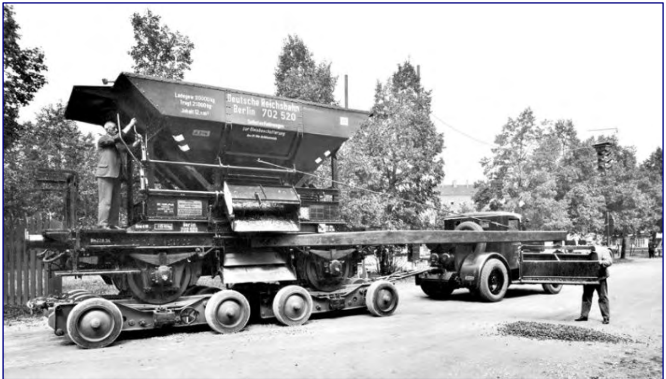
At a road construction exhibition held in Munich in 1934, the 20 t ballast wagon on a road roller demonstrates its basic suitability for road construction when filling in potholes. The Talbot-built self-unloading wagon for track ballasting "Berlin 702 520" is a real classic of railway service wagons. Photo: RVM, Eisenbahnstiftung
