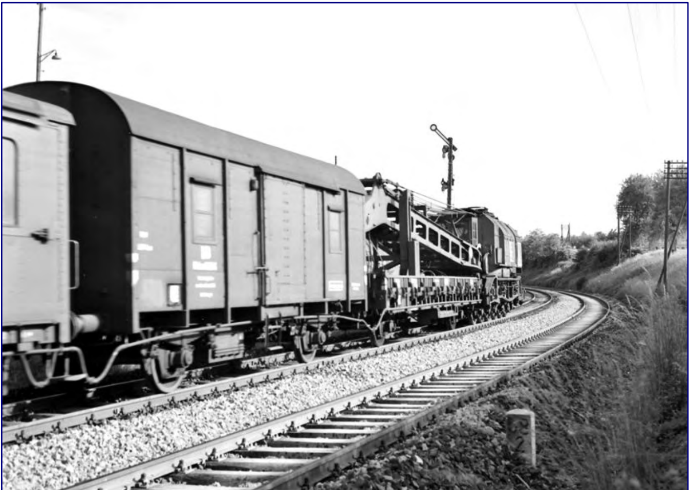
The Ardelt 57 t "Mainz 6600" steam crane is on the way to a job site on June 22, 1968 near Schwäbisch Hall-Hessental. Its jib rests on the "Mainz 6650" crane tender. Photo: Heinz Hangarter, Collection Eisenbahnstiftung
