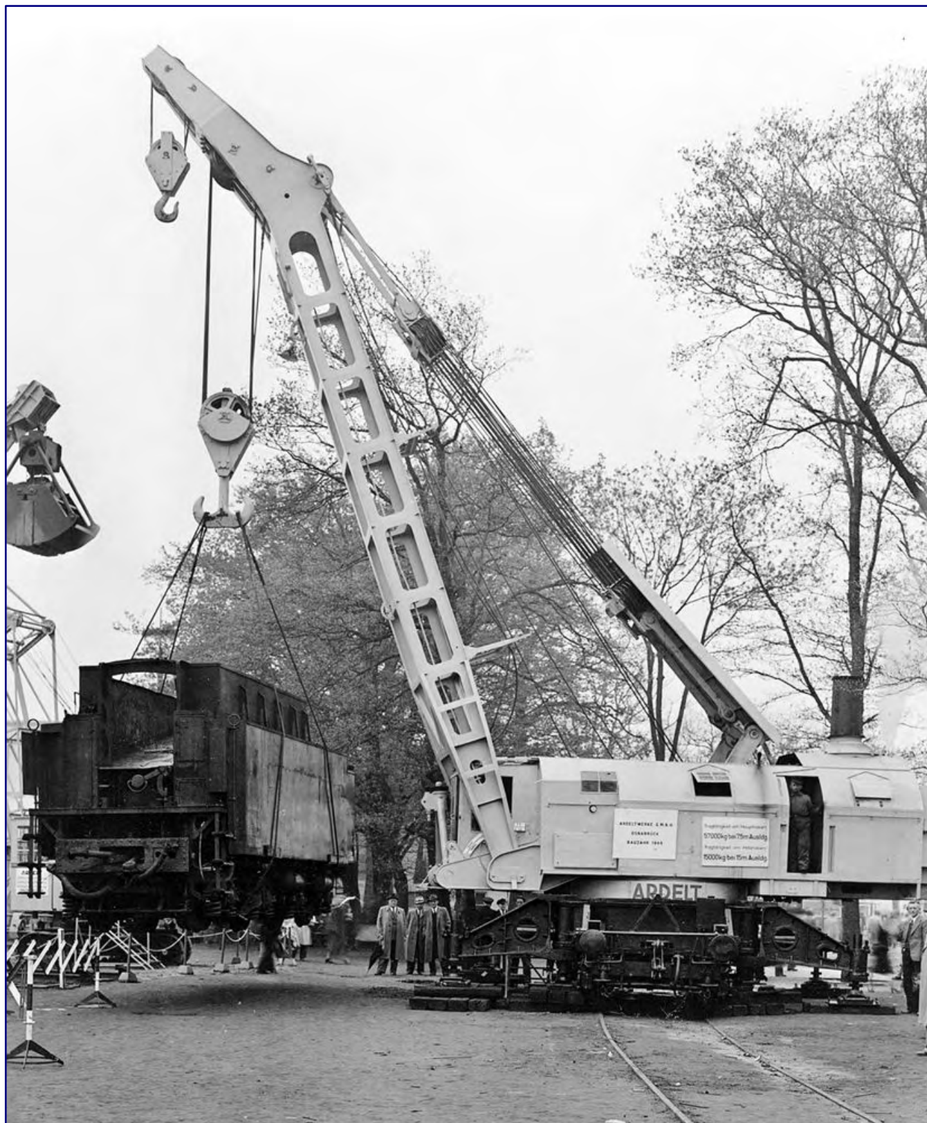
In 1957, Ardel's 57-tonne cranes were still among the most modern lifting equipment the Bundesbahn had to offer. Thus, during a trade fair demonstration, the performance of the apparently golden-yellow painted rail crane is demonstrated on a tender. This was done with a low outreach but maximum support. Interesting for the model to be presented today is the layering of the construction sleepers on which the stabilisers of the supports rest. Photo: Slg. Eisenbahnstiftung
