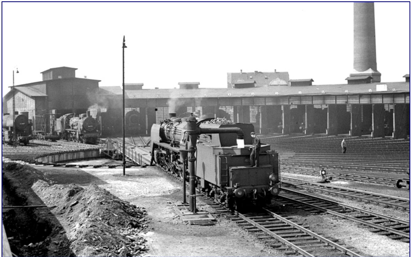
41 010 (Mönchengladbach depot) restored in 1950 at the Duisburg Hbf depot, which was closed in 1966. In the meantime, the steam locomotive has also given up its tender and received a 2'2' T 32 in exchange. 38 3772 and 42 1507 can be seen in the background. Photo: Willi Marotz, Eisenbahnstiftung
