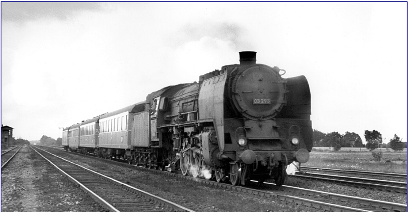
Photo above: On the Cornberg ramp we see 44 1392 (Bw Göttingen Vbf) from DB stock, still equipped with a 2'2" T 32 type tender on 21 April 1961. The open water box lid illustrates the central position, the opening lower down the side is an emergency inlet. Photo: Joachim Claus, Eisenbahnstiftung
