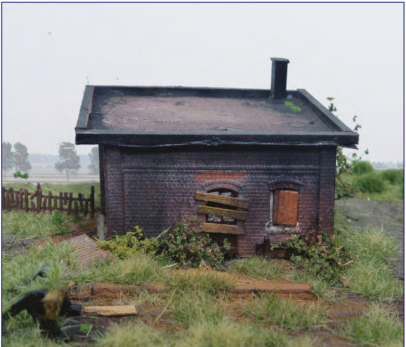
This small and boarded-up building belonged for decades to the steam locomotive depot at the terminal station “Helenensiel.” A piece of track and the buffer stop still exist.
