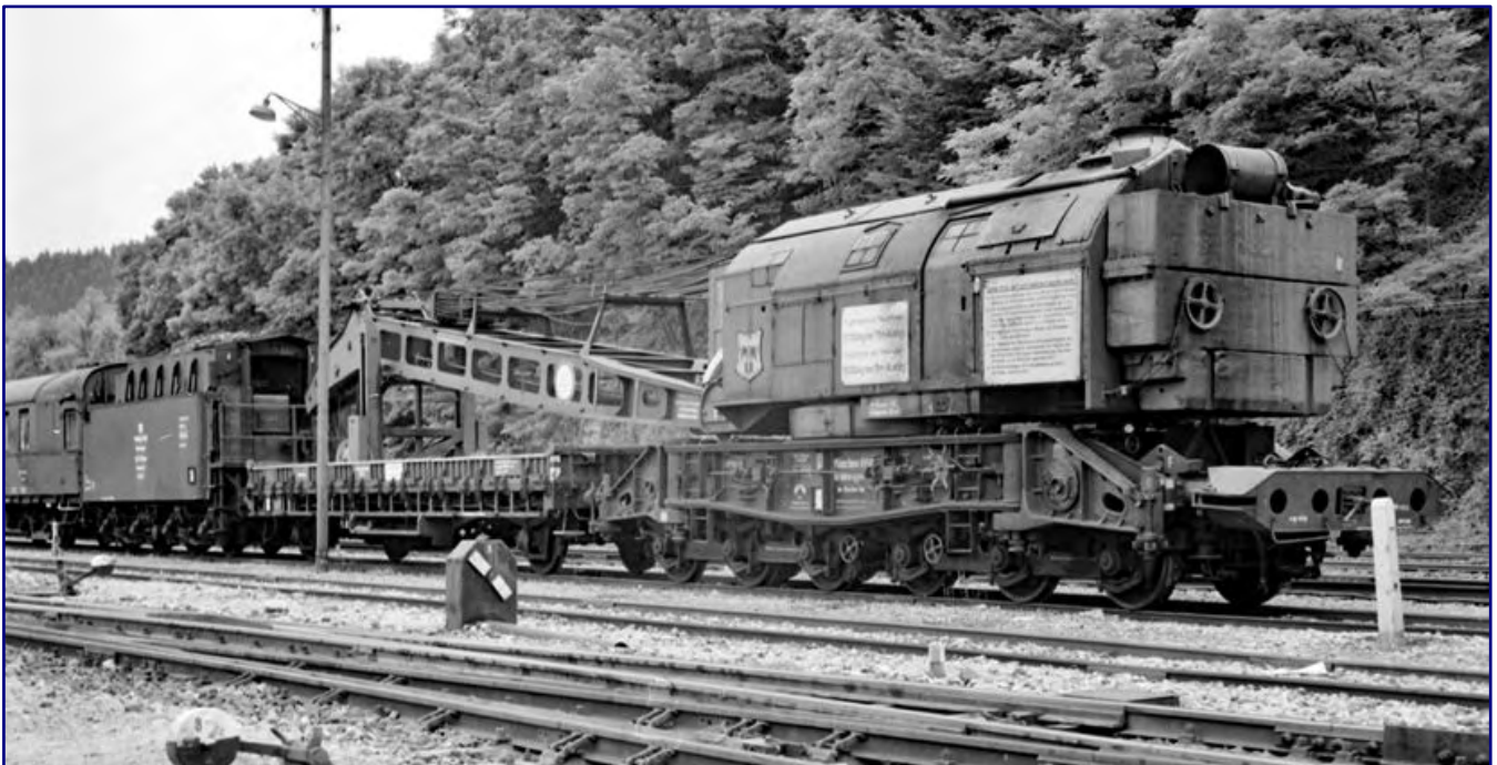
On 13 July 1968, the 57 to. crane “München 6664” stands in Gaildorf-West station to replace bridge parts on the Kocher Bridge. The photo also shows the supplying tender 2'2' T 34 and the staging car for the crane personnel – a former “Hechtwagen”. Photo: Wolf Schneider, Collection Eisenbahnstiftung
