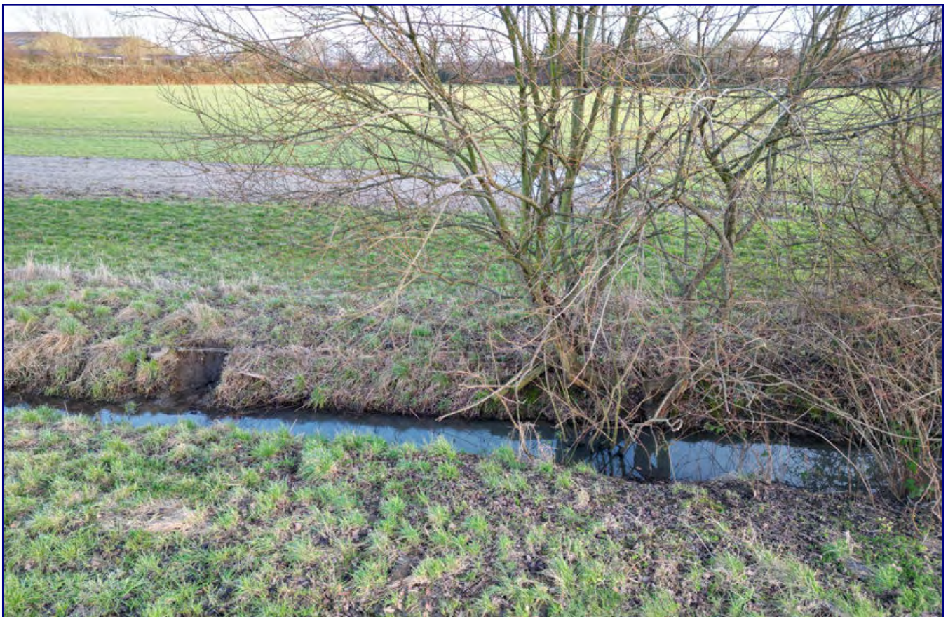
Ditches are man-made and serve to drain water from the landscape. This is why they usually run dead straight, as can be seen here. You can also clearly see that there is a narrow strip without vegetation between the water level and the turf.
