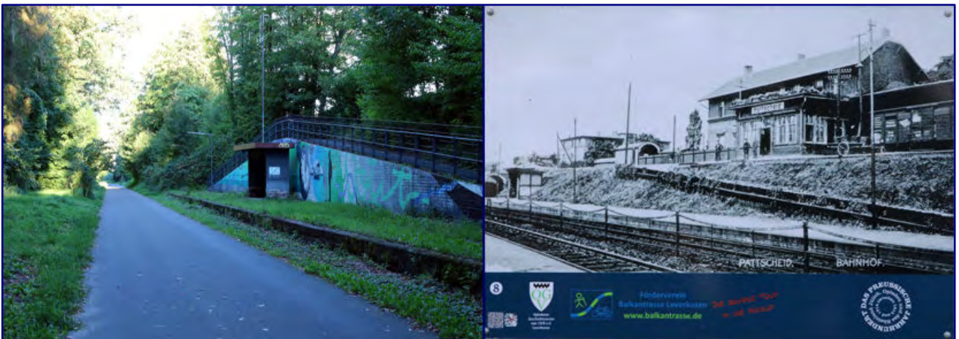
Two views of the exemplary restored Pattscheid station building (photo above). The view of the former track and platform at Pattscheid station in the direction of Opladen can now be seen from a cycle path. A plaque commemorates the original condition (Photo below).
